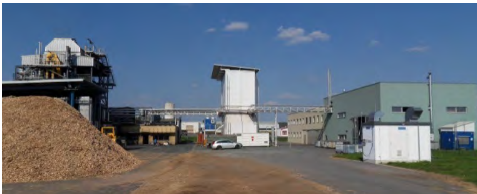
Figure 20. Biomass CHP Güssing (left), BioSNG demonstration plant (middle), Technikum (right) and BioSNG filling station (right front).
