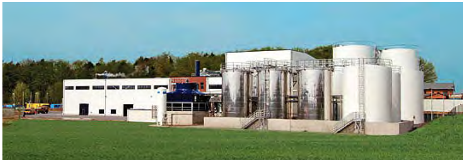
Figure 9. The biodiesel plant Sternberg/Germany.
