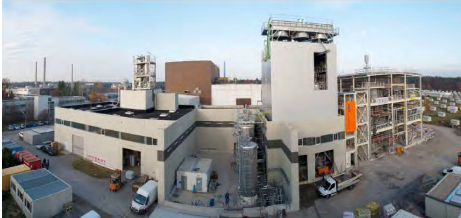
Figure 22. Bioliquid plant under construction.
