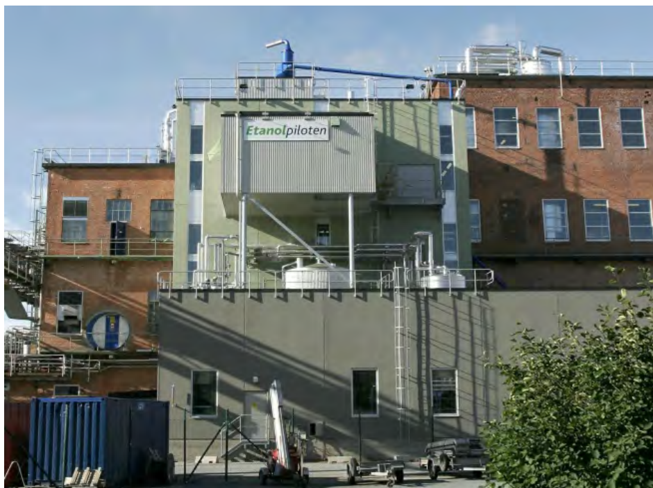
Figure 16. The bioethanol plant in Domsjö/Sweden.
