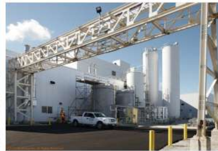
BioAmber's bio-based succinic acid plant in Sarnia, Ont.
