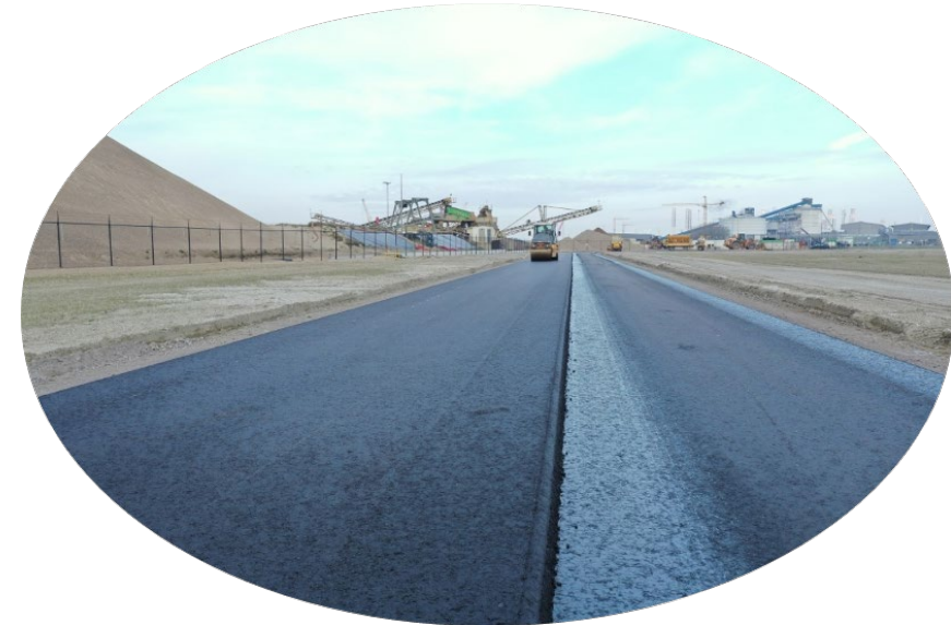
Worlds 1 st 3-layer lignin based asphalt road made by H4A
